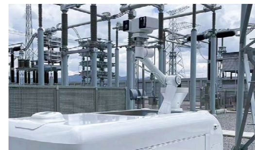
Power plant IR inspection
